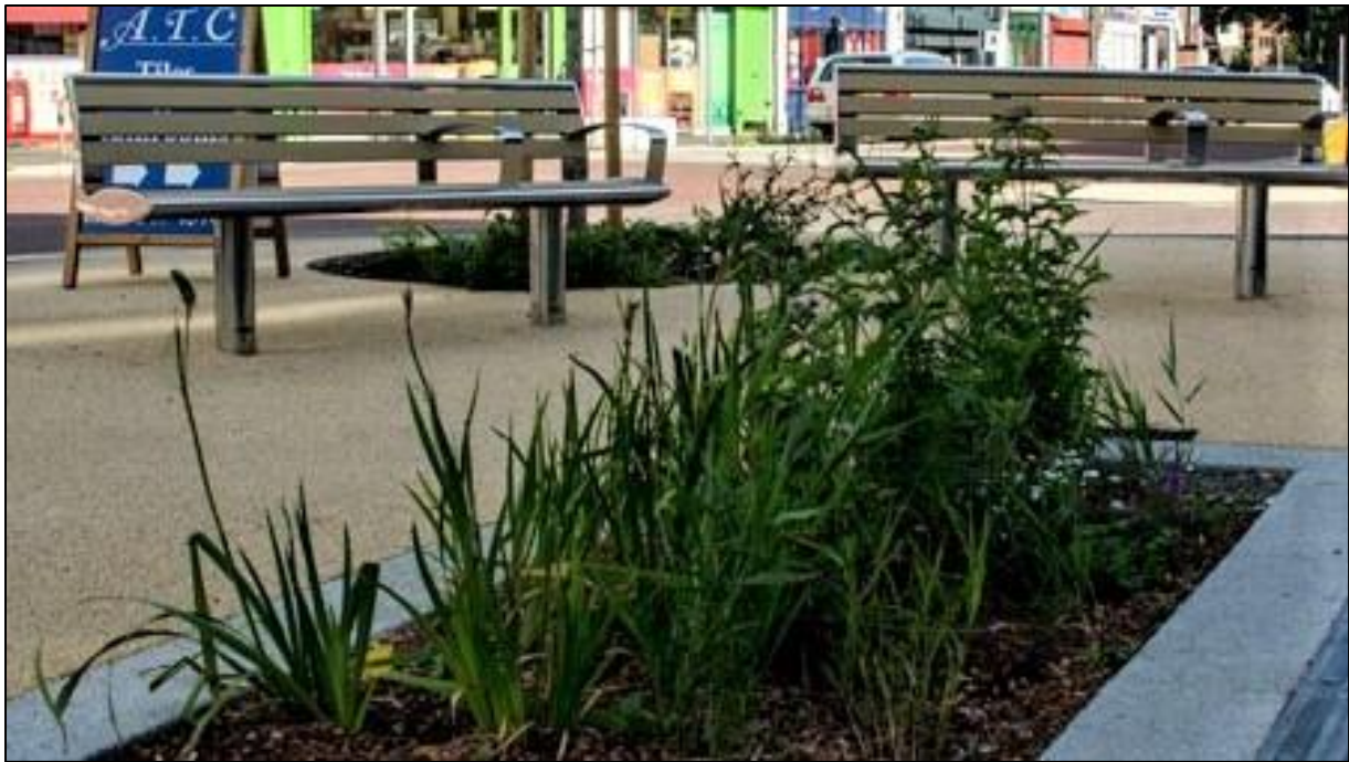
Figure 50: Rain gardens in south London have helped to attenuate urban runoff into the nearby River Wandle. Retrofitting these structures in the urban parts of the catchment could help to reduce scouring flows in the river (Photo: One Planet Sutton).
