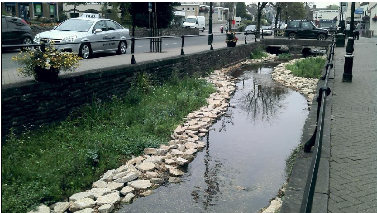
Figure 54: Backfilled and planted rock berms create a meandering channel for the River Somer in its armoured channel through Midsomer Norton, Somerset.
