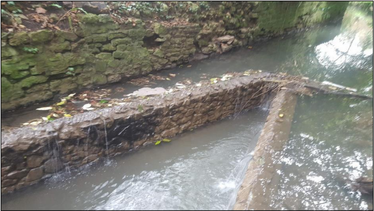
Figure 22: The weir at the upstream extent of the visited section of the Hazel Brook is a barrier to fish passage. The brook shows signs of nutrient enrichment
