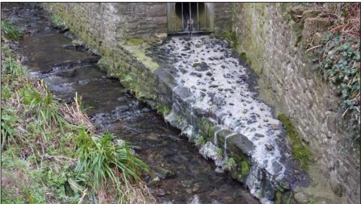
Figure 16: A serious misconnection problem in Westbury.
