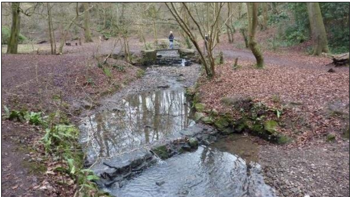
Figure 11: Two of the weirs in Badock's Wood. Possibly installed to 'keep water in the river' in this area of natural sinkholes, they are now doing more ecological harm than good. Removing the weirs and introducing natural woody features would create a healthier and more varied channel structure.
