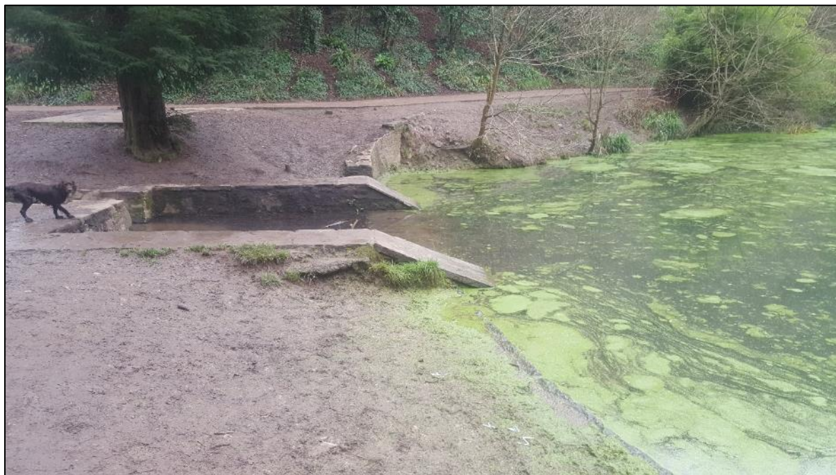
Figure 33: The small sediment trap is not enough to prevent sediment and pollutants accumulating in the pond.
