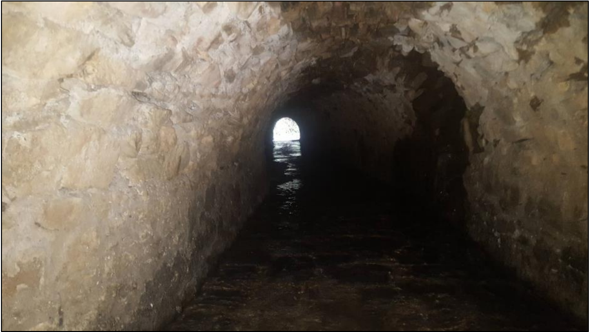
Figure 34: The culvert under the path around the pond is flat-bottomed and a barrier to fish passage
