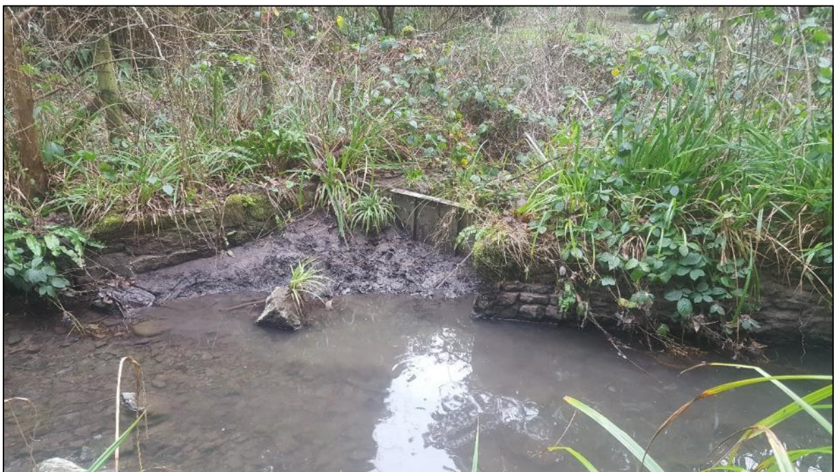
Figure 37: The offtake for the pond is silted up and the pond is offline, suggesting the weir could be removed.
