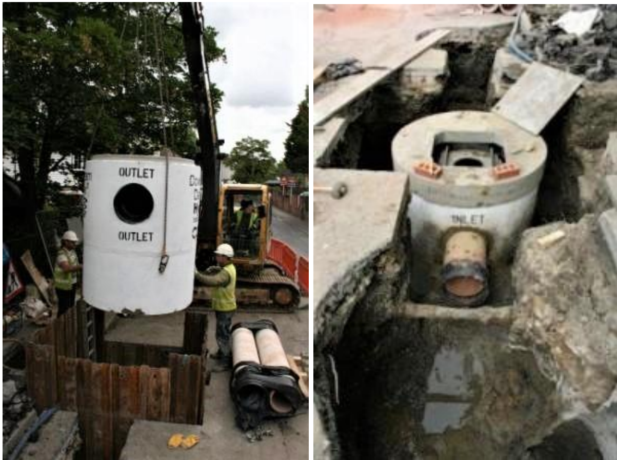
Figure 49: Downstream Defender hydrodynamic vortex chamber silt traps, originally designed for very high volumes of motorway runoff, being installed to intercept sediment in surface water drains in south London (Photo: South East Rivers Trust)
