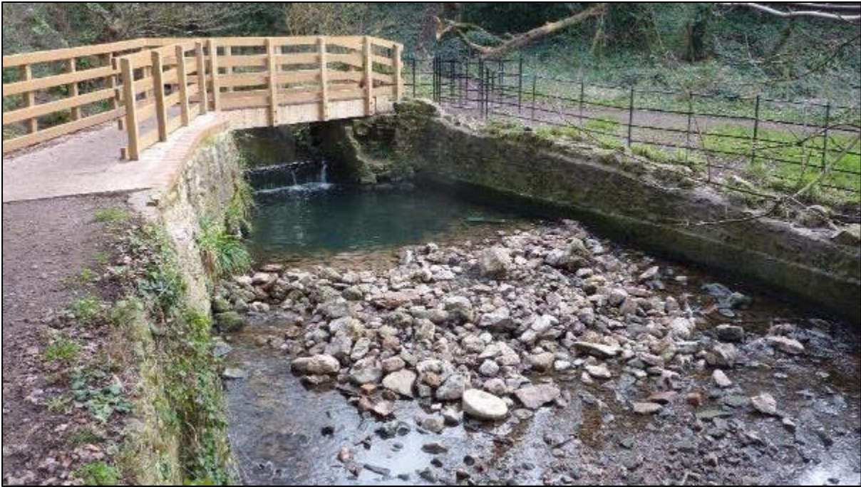
Figure 21: Just before its junction with the Hazel Brook, this weir is a significant barrier to migrating fish.
