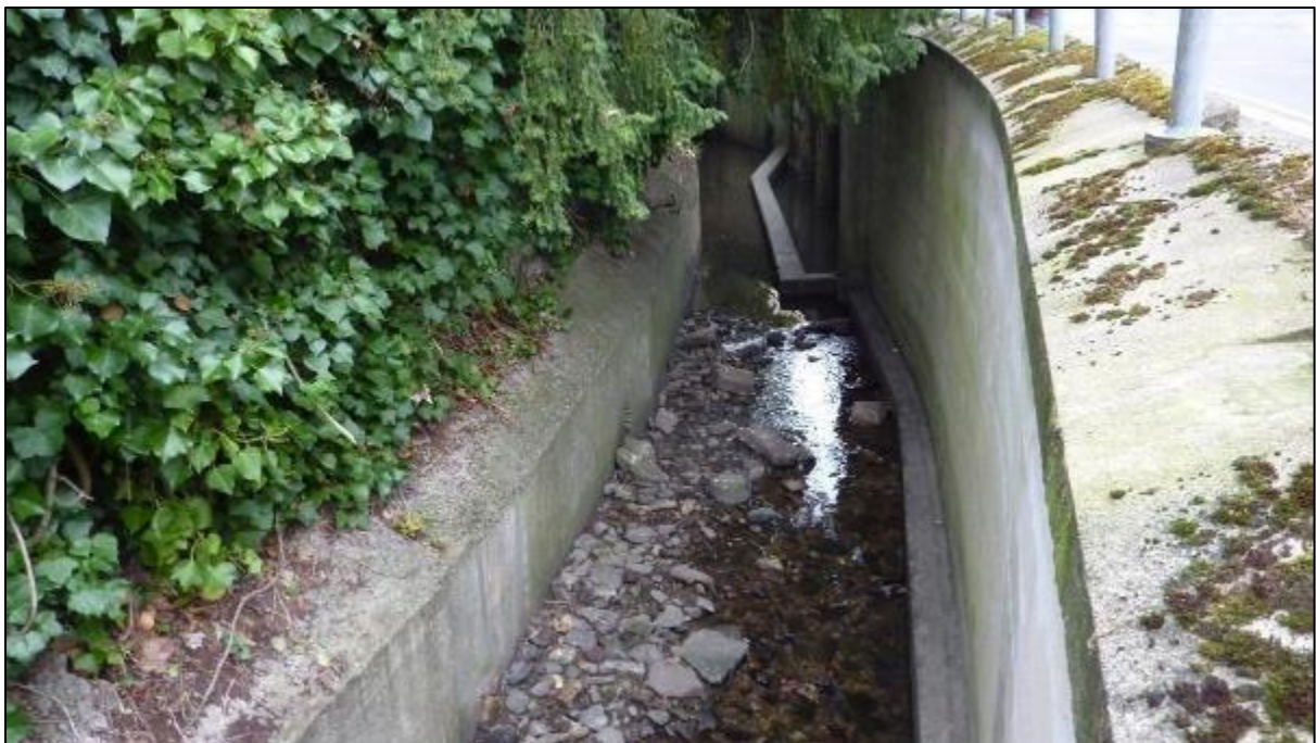
Figure 17: The throttled offtake to Westbury's large underground flood defence scheme.
