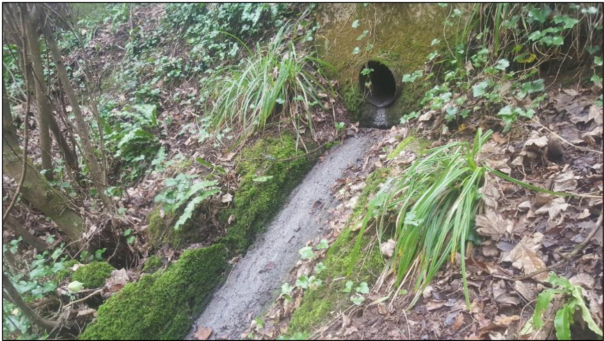
Figure 38: Sewage fungus stains the outfall, suggesting misconnected foul water
