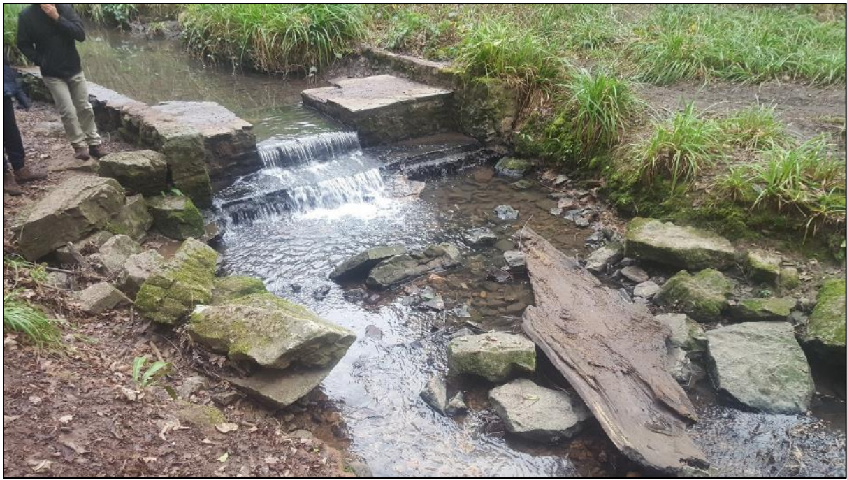
Figure 36: Another weir, presumably constructed to divert flow into the adjacent pond
