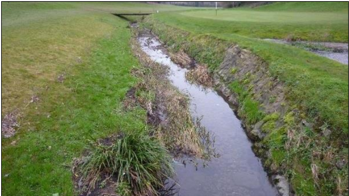
Figure 18: Through Henbury golf course, the Trym's channel has been partly softened with coir rolls on the RB.
