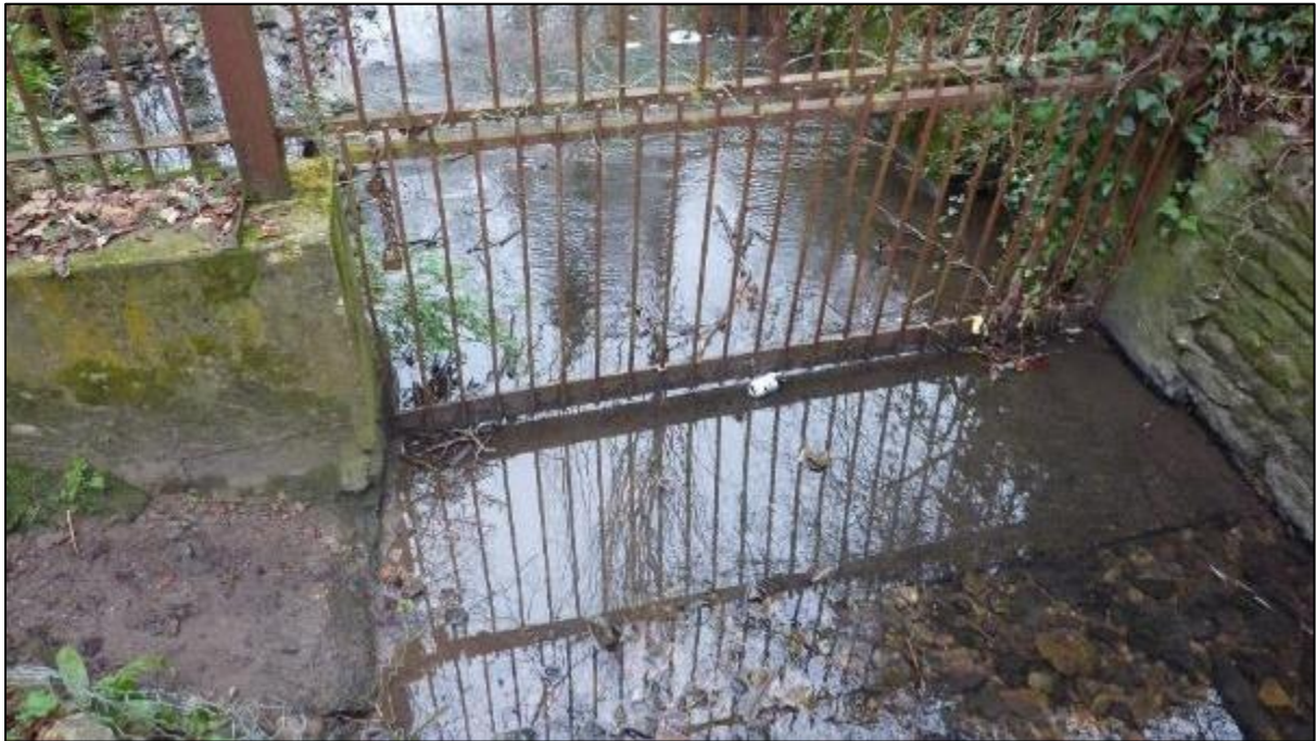
Figure 14: Water gate between Badock's Wood and private land. Removing the concrete sill would restore fish passage and downstream sediment movement at this point.
