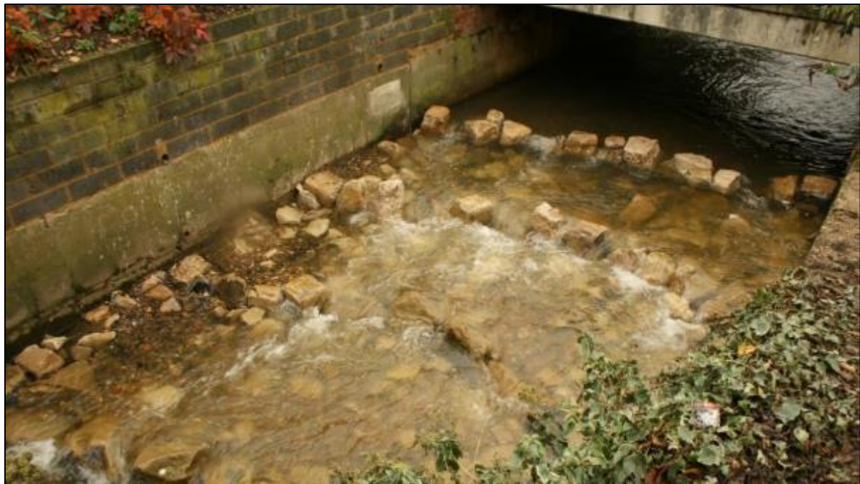
Figure 56: Introduced rocks and gravel create a range of habitats and flow dynamics in what was once a smooth concrete channel in the Hogsmill River (Photo: SERT)
