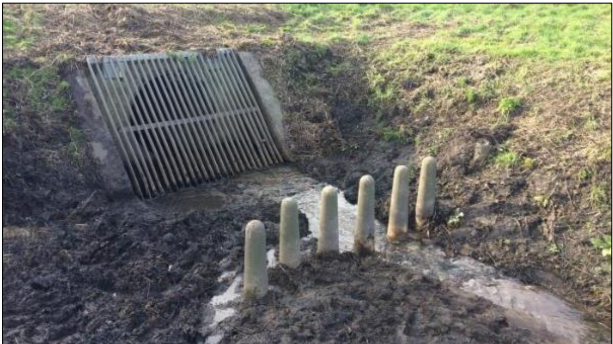
Figure 10: The trash screen over the deep culvert at the lower end of the Southmead green space, after clearance by SusWoT volunteers. The line of concrete bollards was probably installed to stop larger items of fly tipping and other urban debris from blocking the screen after being swept downstream by high runoff. (Photo: SusWoT)
